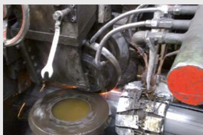
Temperature monitoring of pipe rims shortly before welding
